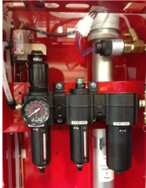
Figure 2: Particulate, Coalescing, and Absorber, respectively
