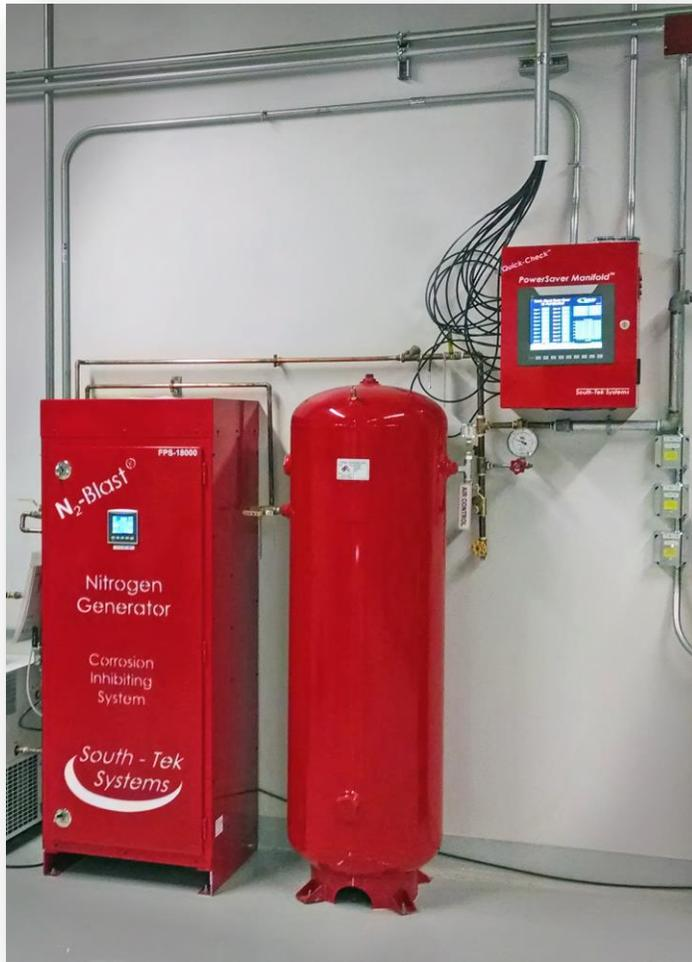
This nitrogen generating system, which protects multiple fire protection systems in one building, consists of the nitrogen generator (left), the nitrogen gas receiver tank (center), and a control panel (right) that monitors the nitrogen purity concentration within the multiple pre-action systems. Photo courtesy of South-Tek Systems.
