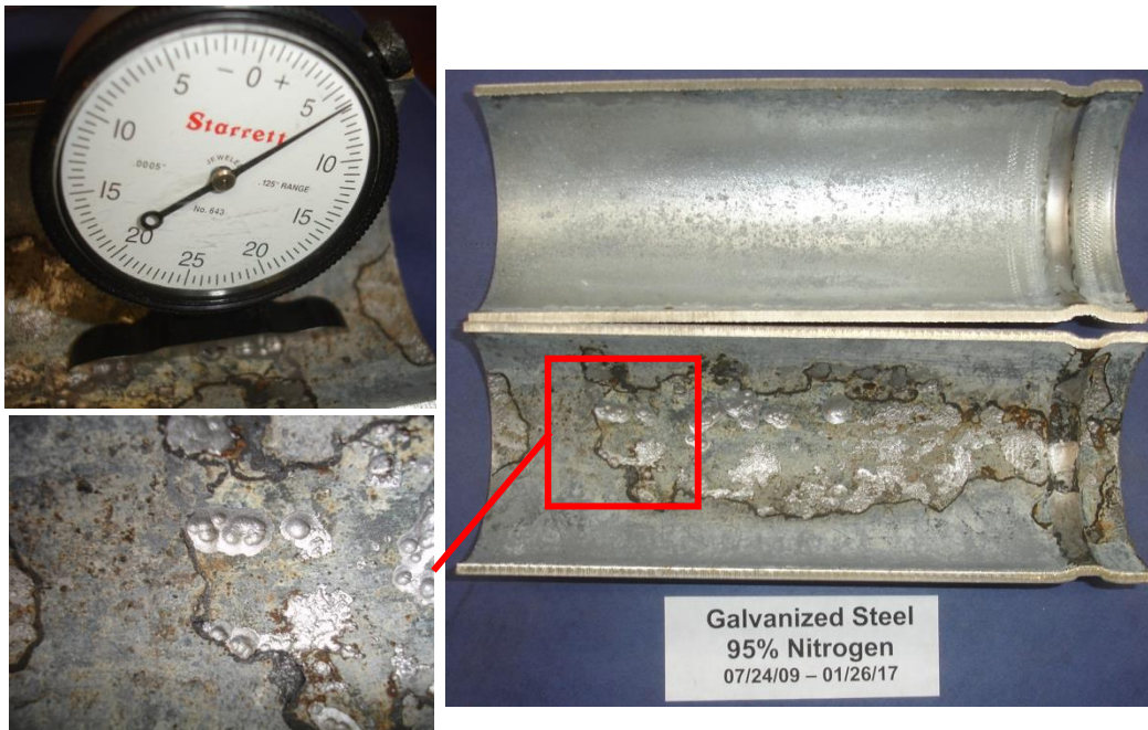
Figure 10. Composite image of cleaned galvanized piping after 2893 days of exposure while half-filled with water and under 95% nitrogen supervision. Note the presence of localized pits in areas where zinc coating is no longer present
