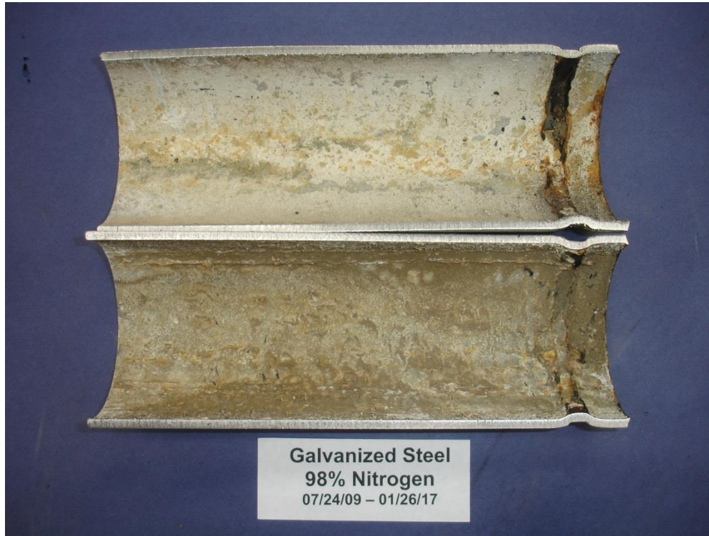
Figure 7. As found condition of interior surface of galvanized steel piping after 2893 days of exposure while half-filled with water and under 98% nitrogen supervision.
