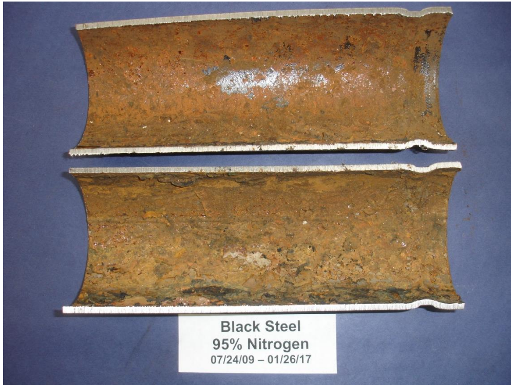
Figure 3. As found condition of interior surface of black steel piping after 2893 days of exposure while half-filled with water and under 95% nitrogen supervision.
