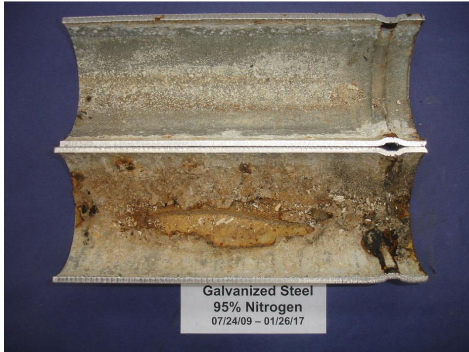
Figure 9. As found condition of interior surface of galvanized steel piping after 2893 days of exposure while half-filled with water and under 95% nitrogen supervision.
