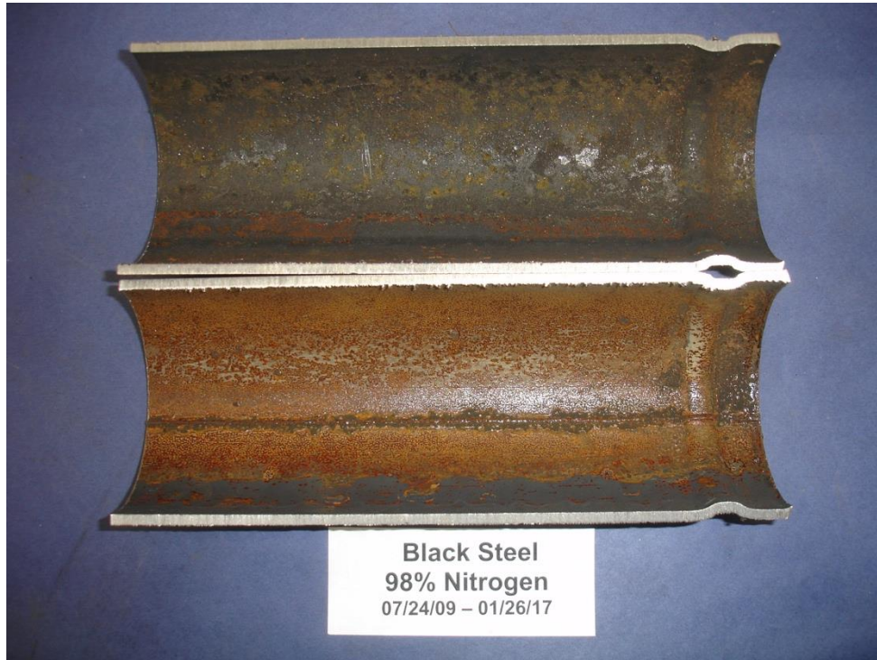
Figure 5. As found condition of interior surface of black steel piping after 2893 days of exposure while half-filled with water and under 98% nitrogen supervision.
