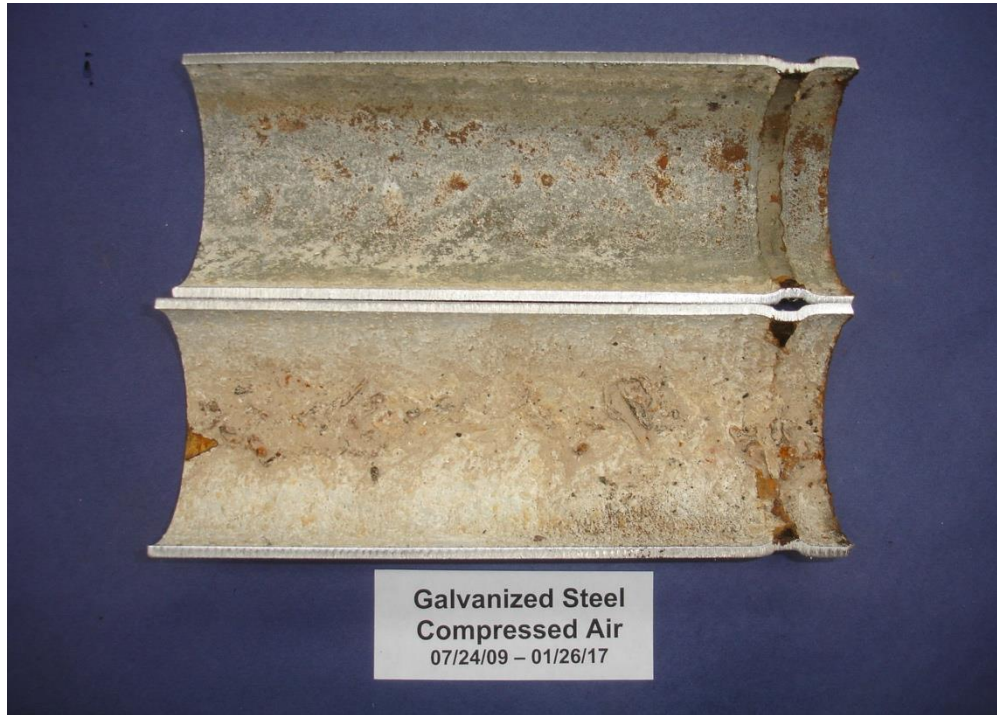
Figure 7. As found condition of interior surface of galvanized steel piping after 2893 days of exposure while half-filled with water and under compressed air supervision.
