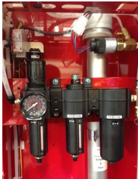
Figure 2: Particulate, Coalescing, and Absorber, respectively
