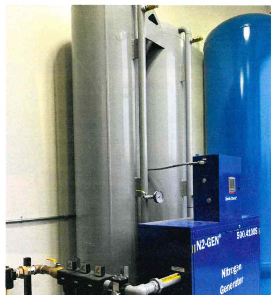
A pressure swing adsorption nitrogen generator can be tuned to meet the purity and flow rate requirements a fabricator needs. Photo courtesy of South-Tek Systems.
