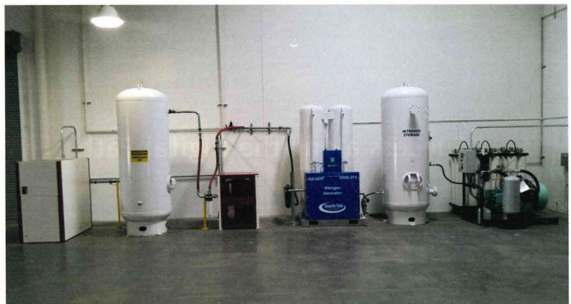
A 16-pack bank of high-pressure cylinders (on right) serve as a buffer, allowing the nitrogen generation system to adapt to varying levels of demand.
