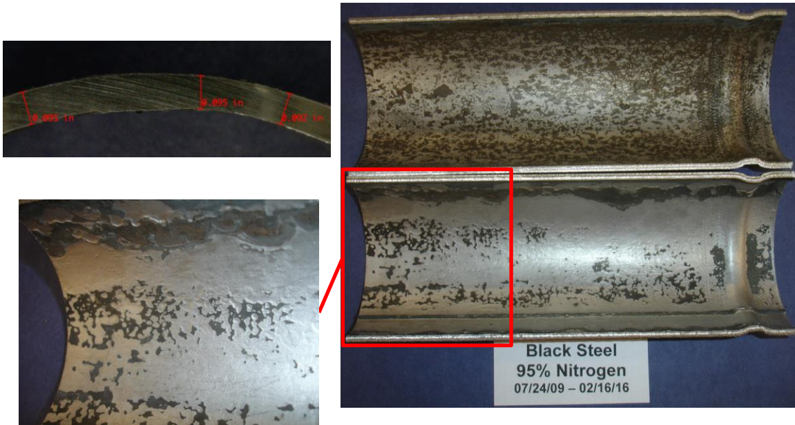
Figure 3. Composite image of cleaned black steel piping after 2398 days exposure while half-filled with water and under 95% nitrogen supervision. Note uniform appearance of pipe wall and absence of any localized pits.
