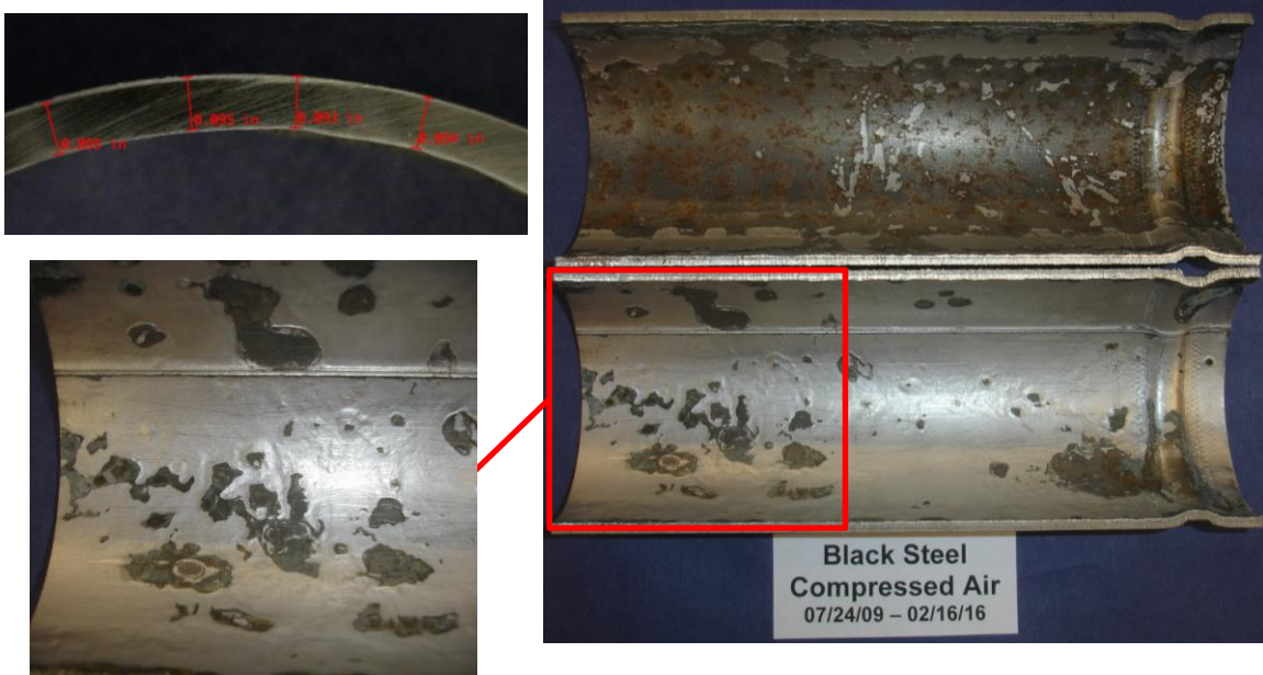
Figure 1. Composite image of cleaned black steel piping after 2398 days exposure while half-filled with water and under compressed air supervision. Note uniform thinning of pipe wall with a few localized, shallow pits.
