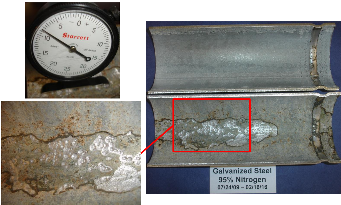
Figure 4. Composite image of cleaned galvanized piping after 2398 days exposure while half-filled with water and under 95% nitrogen supervision. Note the presence of localized pits in areas where zinc coating is no longer present.
