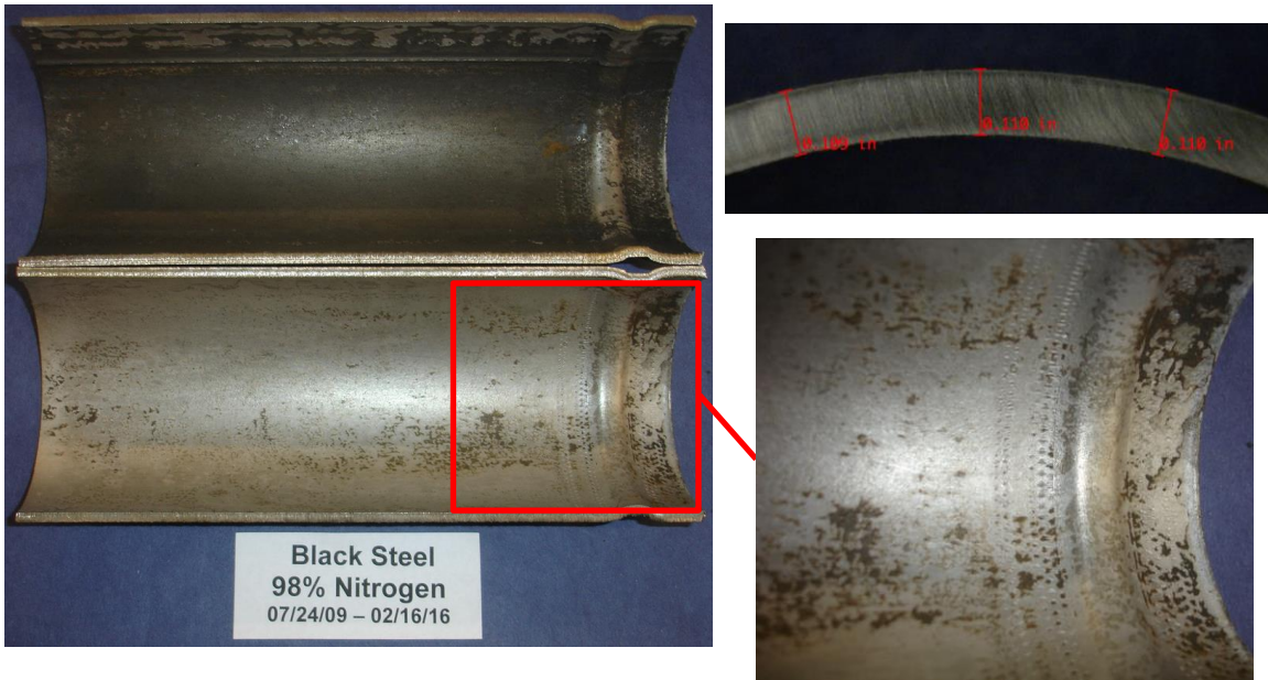
Figure 5. Composite image of cleaned black steel piping after 2398 days exposure while half-filled with water and under 98% nitrogen supervision. Note uniform appearance of pipe wall and absence of any localized pits.
