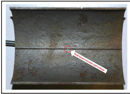
Figure 3. Photograph showing preferential grooving corrosion on pipe weld seam with a 1 mm pinhole leakage inside a black steel pipe (NPS 3, schedule 10).
