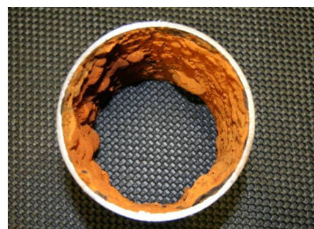
Figure 2. Photograph showing tubercles heavily formed inside a black steel sprinkler pipe (NPS 4, schedule 10).
