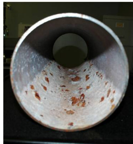
Figure 1. Photograph showing corrosion of galvanized steel pipe (NPS 6, schedule 10) where residual water filled about 40 percent of the pipe’s volume in a pre-action system.
